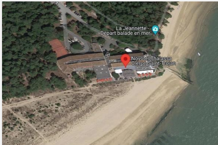
Novotel Oleron Saint Trojan Description
