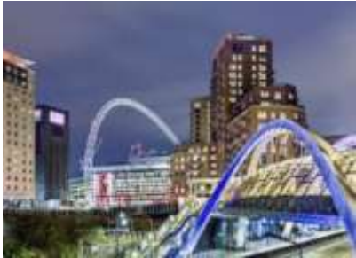
IBIS Wembley Refurbishment
