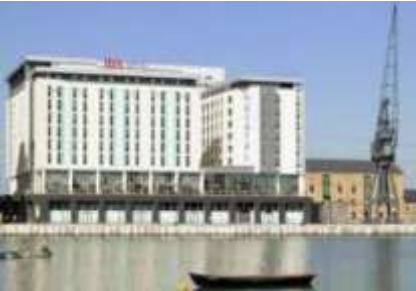
IBIS Excel Refurbishment
