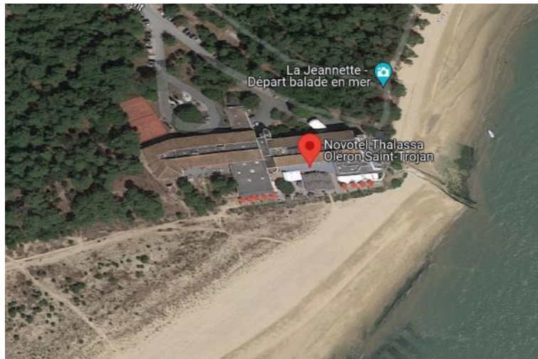
Novotel Oleron Saint Trojan Description
